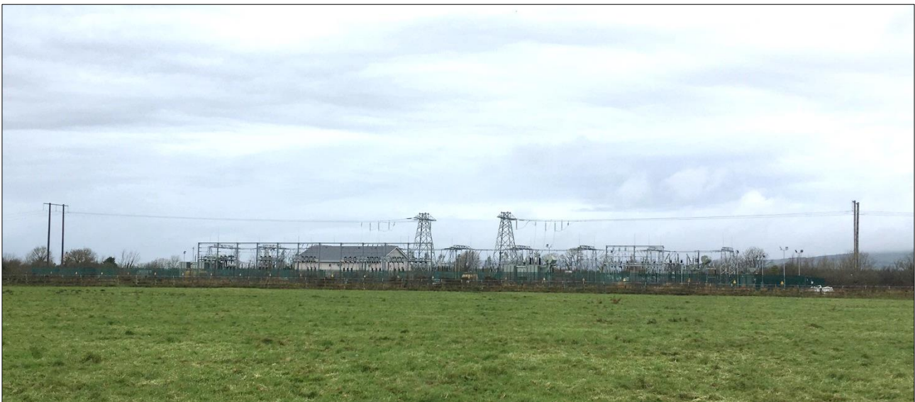
Plate 5-1: Example of similar 110kV substation with End Masts connecting to overhead 110kV line
