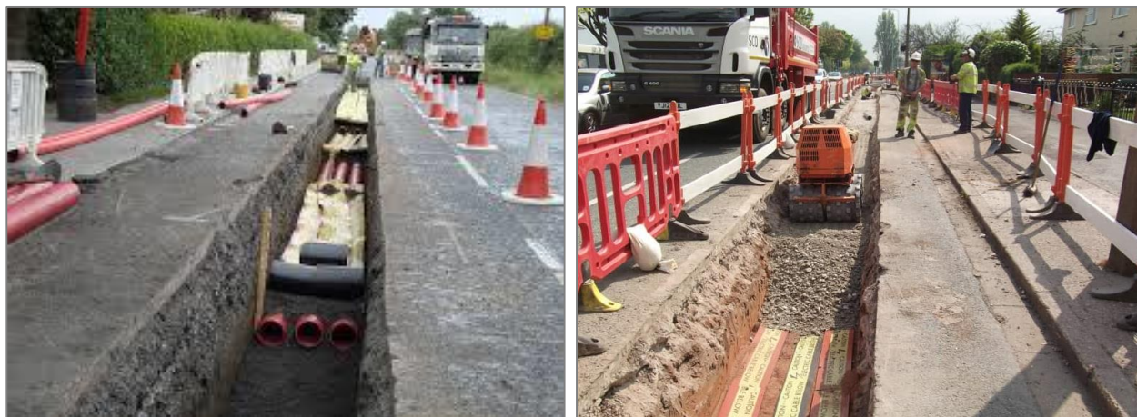
Plate 5-2: Typical Trenching Works set-up on the Public Road
